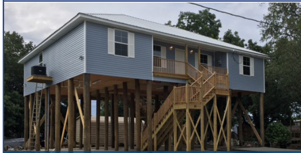
HOME RECONSTRUCTION WITH ELEVATION
