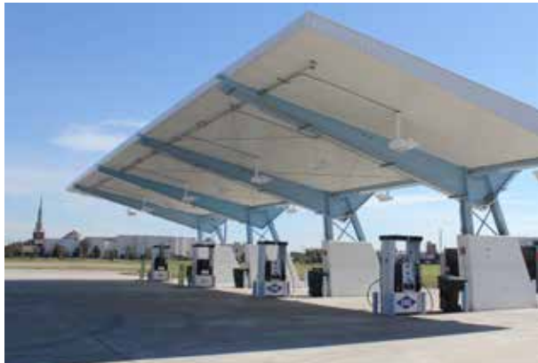
City of Bossier: CNG Fueling Facility.
